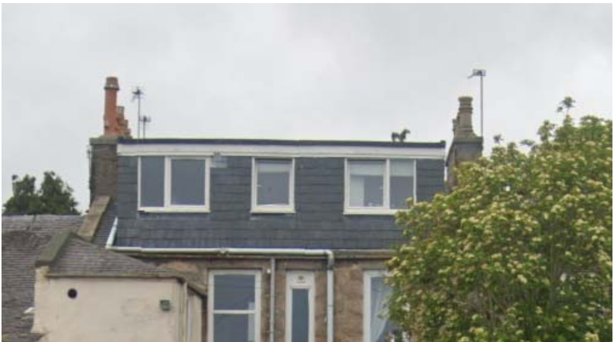
Existing example in the street, viewed from private road.
