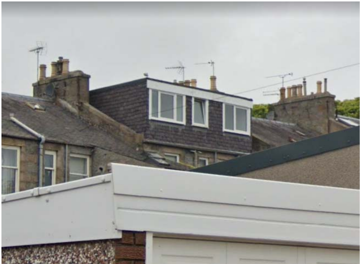
Existing example in the street, viewed from private road.
