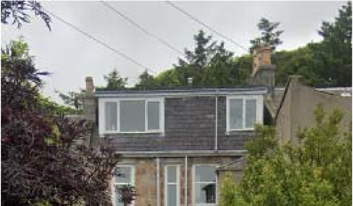
Existing example in the street, viewed from private road.
